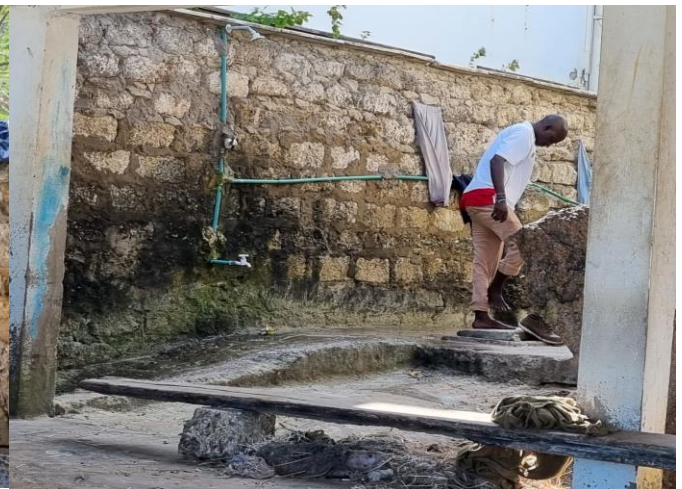
Plate 4-27: Second Shower located near the Fish gear mending shed
