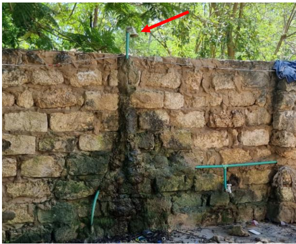
Plate 4-26: One of the Showering point near the existing Toilets
