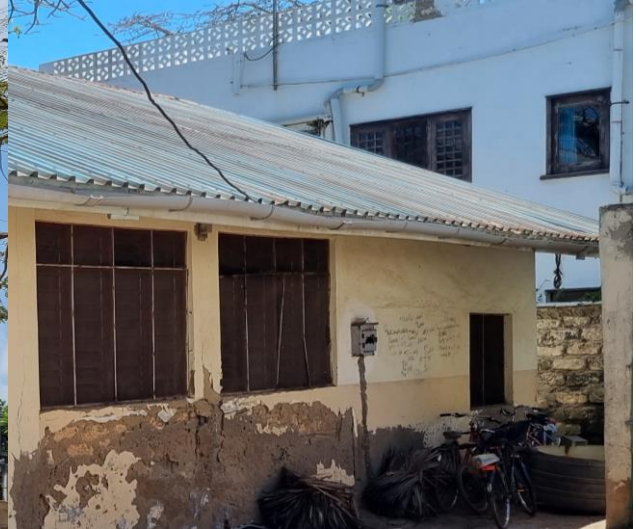
Plate 4-29: The existing Fish Banda Connected to Electricity
