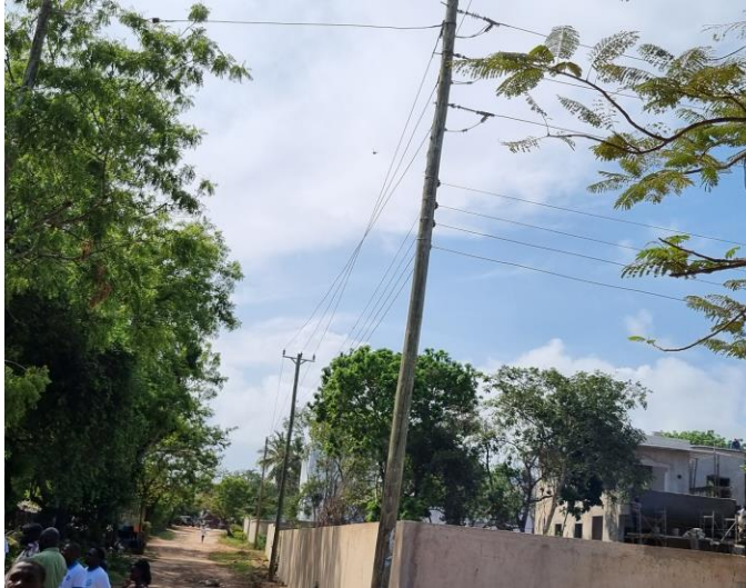
Plate 4-28: Power grid within the project site
