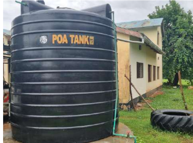
Plate 4-12: Water storage and rain water Harvesting facilities in the project area
