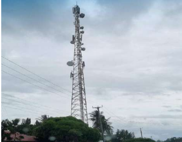
Plate 4-7: Communication Mast for Safaricom
