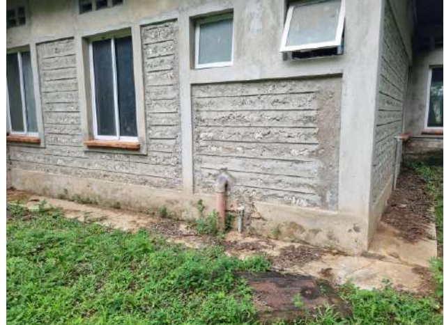
Plate 4-14: Connection of the existing offices in the plot to a septic Tank
