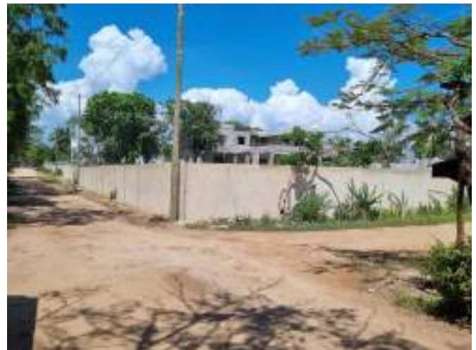
Plate 4-11: A residential House Under Construction Along Mwaepo Landing site Access road
