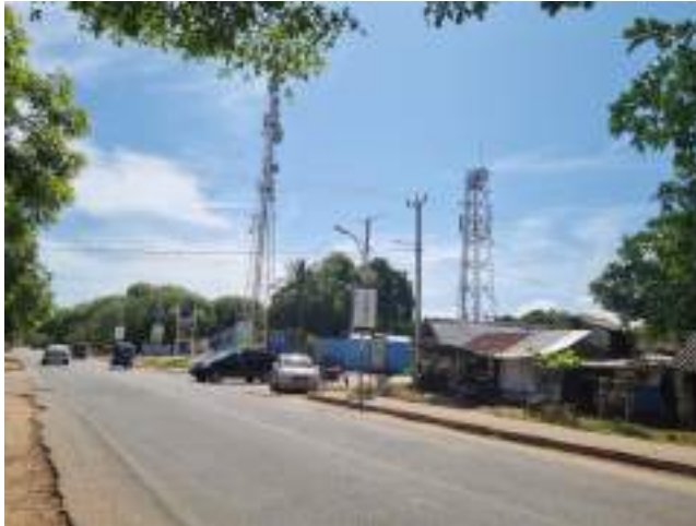
Plate 4-18: Some of the Communication masts Along Diani Beach road
