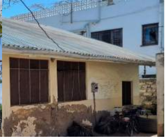
Plate 4-29: The existing Fish Banda Connected to Electricity
