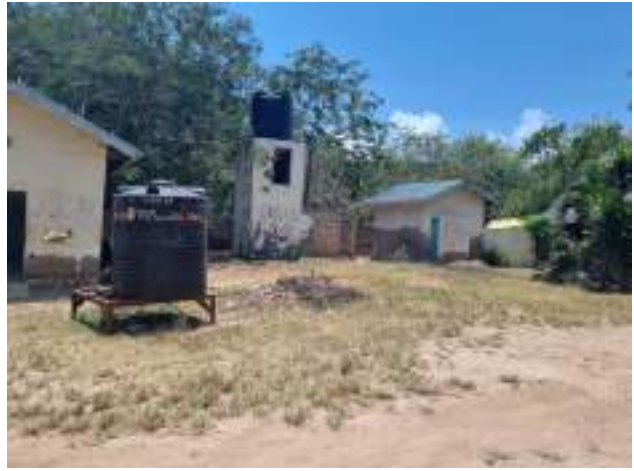
Plate 4-23: Part of the existing water storage facilities at the site
