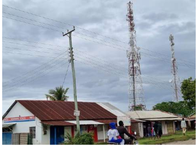
Plate 4-8: Communication Mast for Telecom
