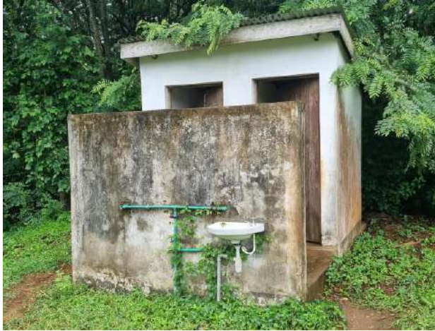
Plate 4-13: One of the Pit Latrines seen in the Area
